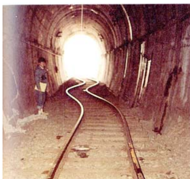
Railway Tunnel which Earthquake Fault passed
