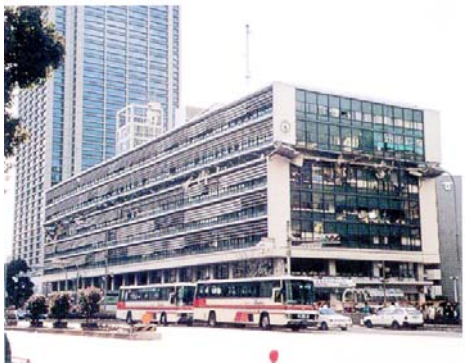
Collapse of Middle Floor
