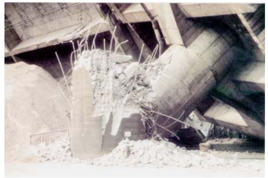
One Column Highway Bridge
