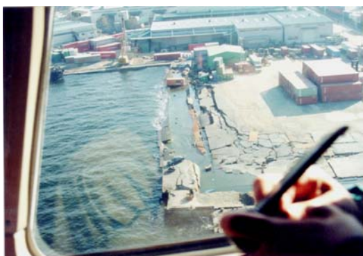
Side Slip of Pier
