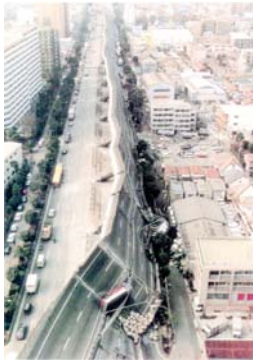
One Column Highway Bridge
