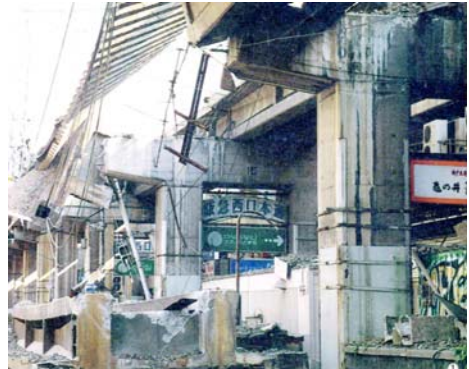
Rail Road Bridge
