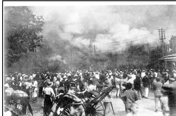
FIRE AFTER EARTHQUAKE
