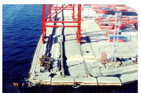
Side Slip of Pier
